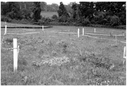
Primary and replacement absorption areas in an open space area. They have been staked, surveyed, and cordoned off so the area is not disturbed until the system is installed. area containing suitable soils for a replacement absorption area nearby.
