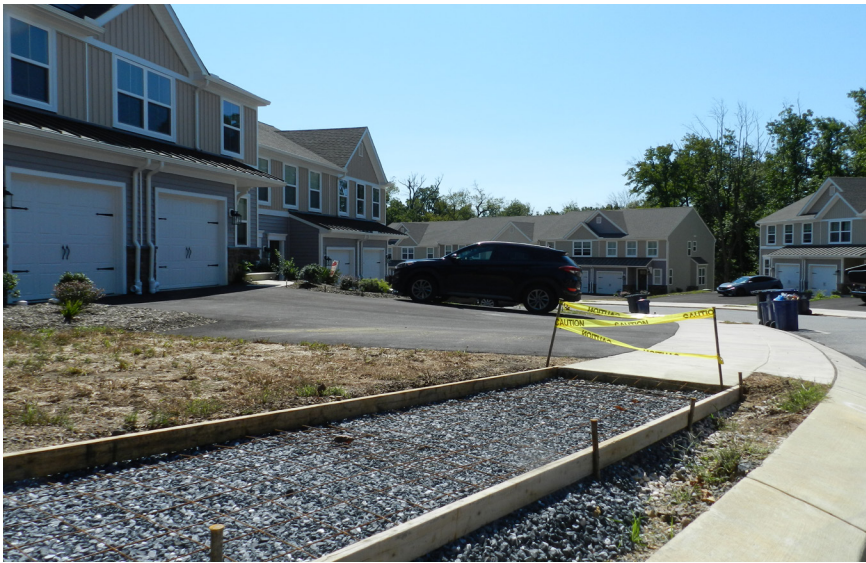
New sidewalks being constructed as part of the Blue Rocks subdivision.
