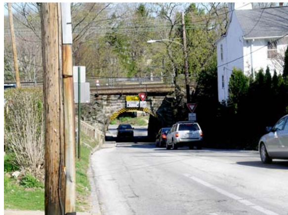
Photo 4.28: Warren Avenue Underpass Looking north along Warren Avenue toward the SEPTA R-5/Amtrak bridge over Warren Avenue. There is a narrow sidewalk on the west side (to the left) of Warren Avenue under the bridge. However, the low arch of the tunnel complicates walking on this particular section sidewalk.
