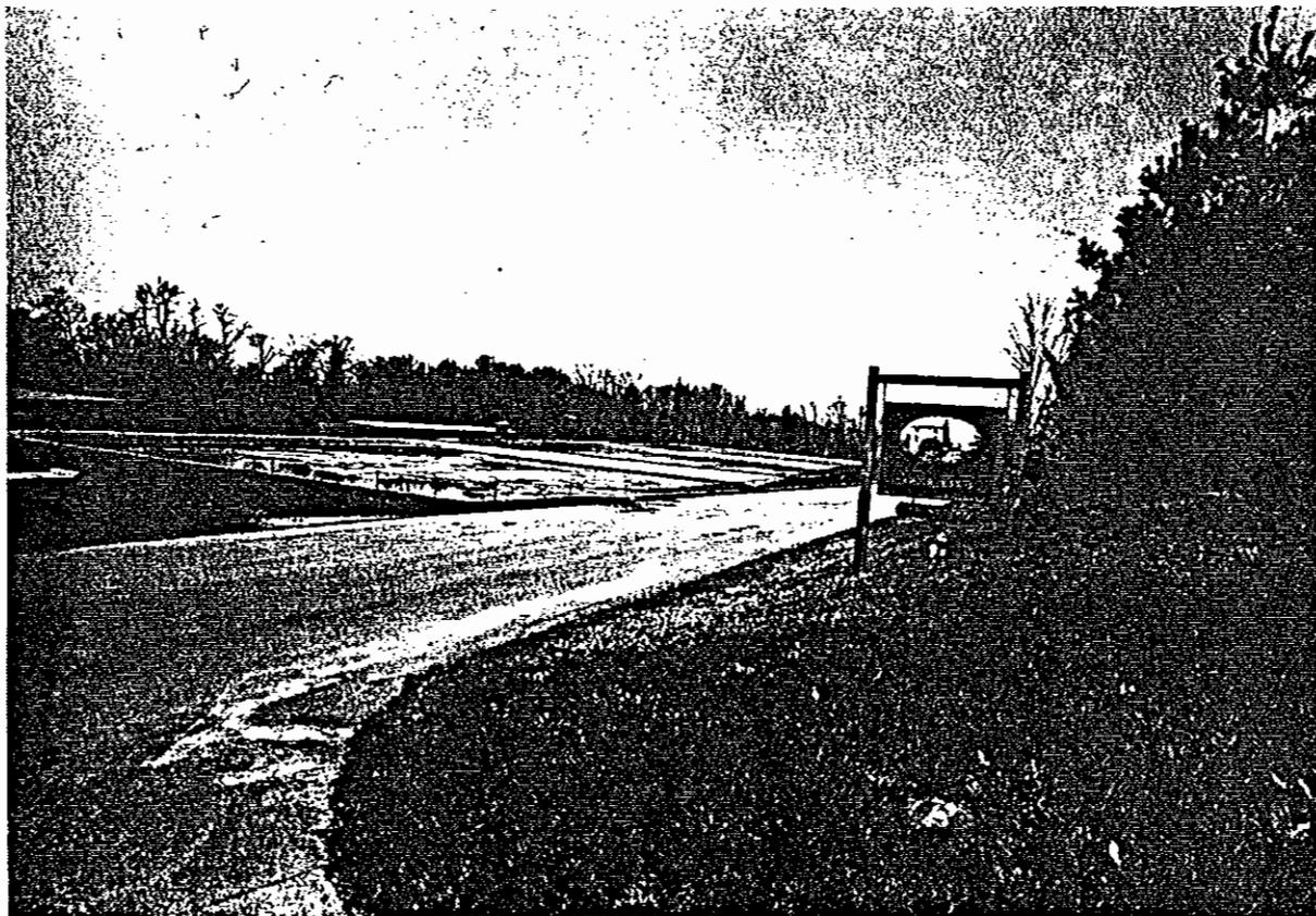
A 26 million gallon storage pond was also constructed. The pond serves two purposes: it stores pretreated wastewater when land treatment is suspended, and it also accepts stormwater during periods of high flow. The latter is accomplished by an intake pipe which, during storm events, can withdraw water in excess of the base stream flow from Ridley Creek.
