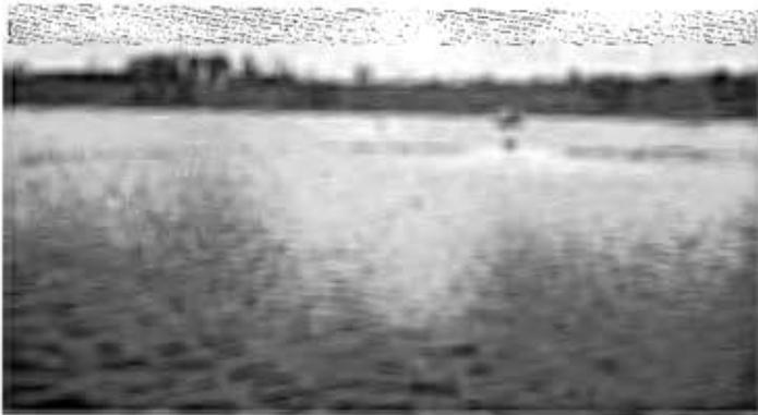
*Aerators in Oxford's primary treatment lagoon add oxygen to the wastewater. Quantity of oxygen added (i.e., amount of aeration) varies directly with how much waste must be treated or "digested."*
