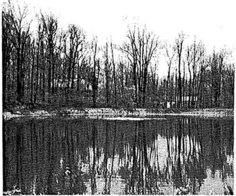
*The aerated lagoons at Lockwood Chase give the appearance of farm ponds. Aerators promote aerobic digestion of waste which, in turn, prevents odor from occurring.*
