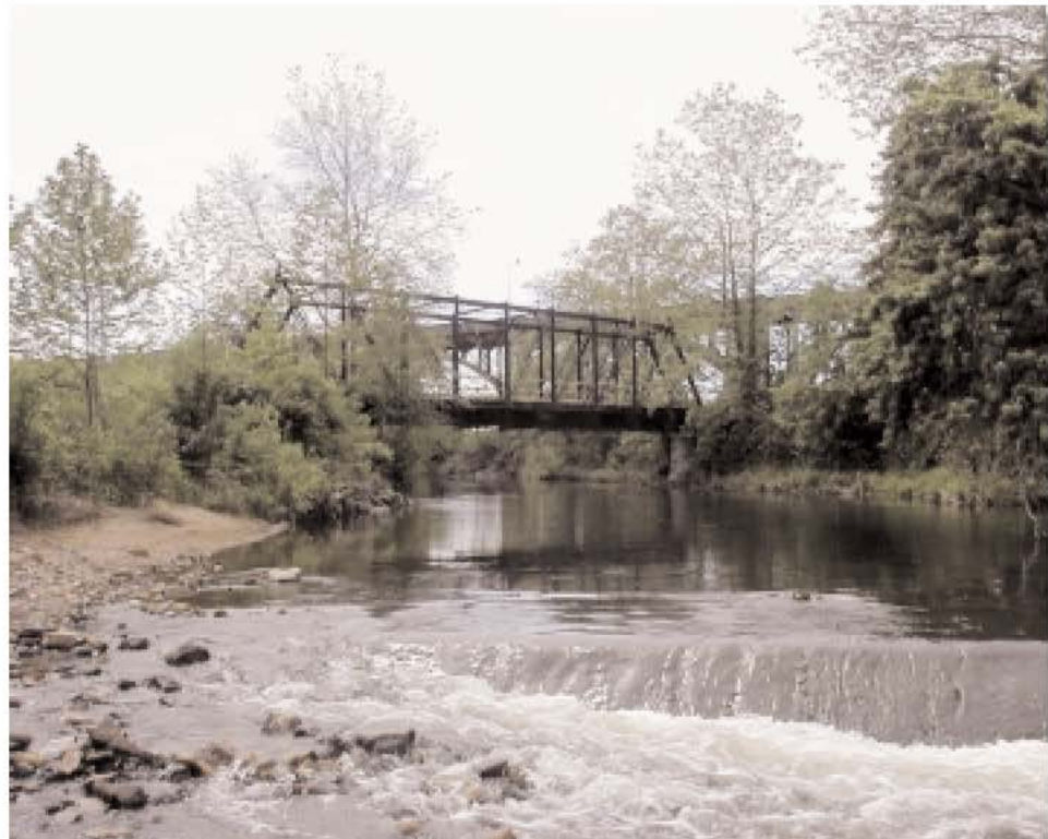
Figure 14.7: The Phoenix Column Bridge across French Creek
