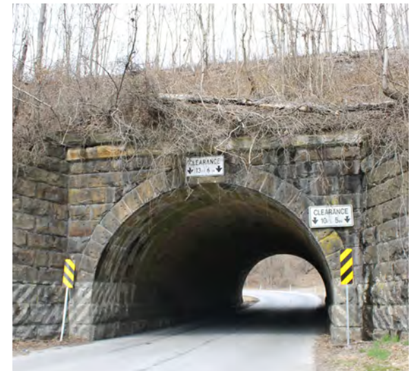
Valley Avenue/Route 372 passes under the Enola Low Grade corridor via this narrow stone arch bridge. Horizontal curvature of the road restrict sight distances at the bridge.
