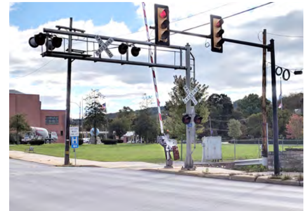
Existing automatic gate does not block pedestrians on the sidewalk from crossing the tracks when a train is coming.
