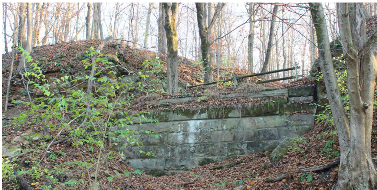
Abutment of a former overhead bridge located in between Southwind Lane and Skelp Level Road.
