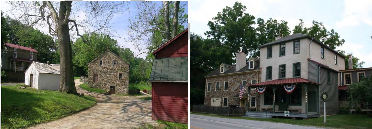
Small non-profit historic sites such as The Mill at Anselma (left) and Historic Sugartown (right) struggle to fund maintenance and visitor improvements and would benefit from a Preservation & Enhancement Program.
