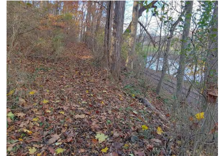
The 1730 Road trace, former section of later realigned to become modern Brinton’s Bridge Rd., west of the Creek. The 18th century roadbed and alignment is still evident as is the narrow cartway.
