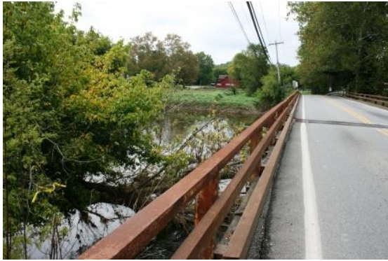
The bridge at this ford site has narrow shoulders.
