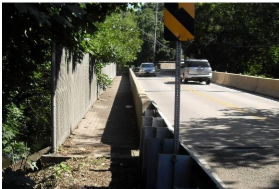
There is sidewalk on half of the bridge's north side.
