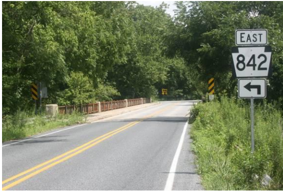
There is a sidewalk on the north side of the bridge.
