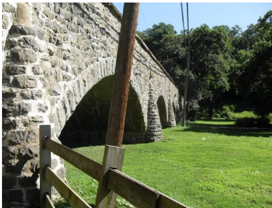
Most of the bridge spans across the floodplain.
