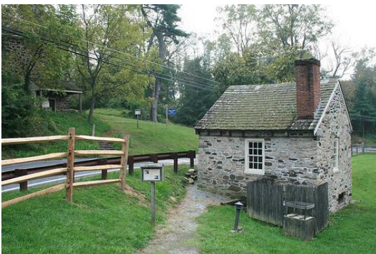
Many historic structures, such as this outbuilding near the John Chad’s House, are close to roads or modern developments that are still actively used.
