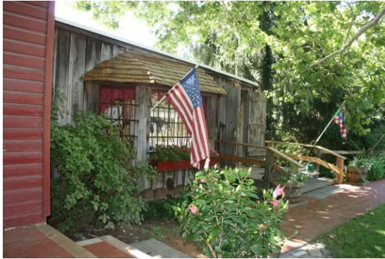
Strode's Mills is a historic structure that is part of the modern landscapes. The building's Battlefield significance is not well known to the public.
