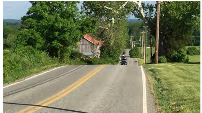
Example of poor roadway alignment.
