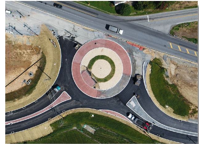
Drone photo of the PA 41 / PA 926 roundabout under construction.
