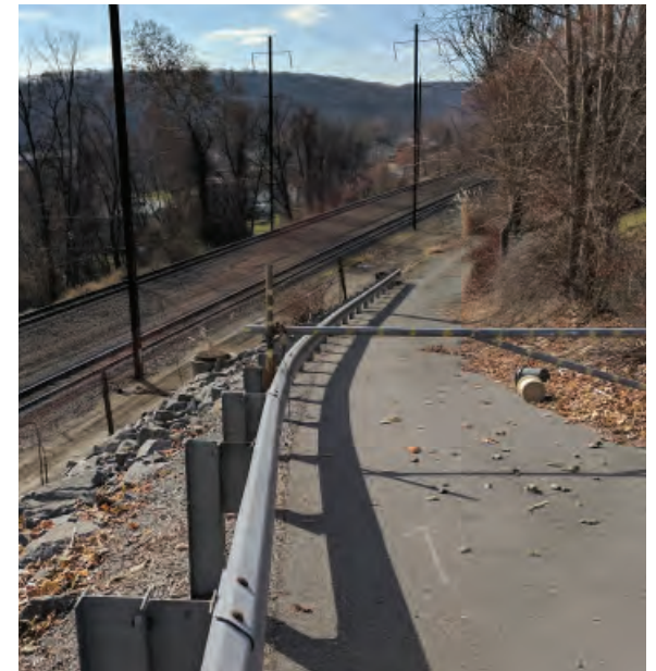
Steep service road leading to Amtrak corridor
