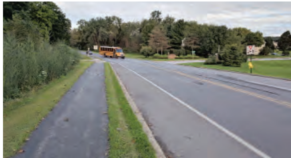
The topography along the existing path drops off toward an adjacent stream. To widen the path, it must be widened toward the roadway.
