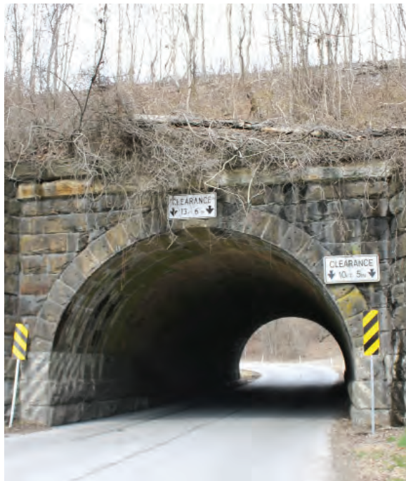
Valley Avenue passes under the Enola Low Grade at this stone arch overpass. The narrow width and minimal sight distance make this portion of the road an undesirable trail route.
