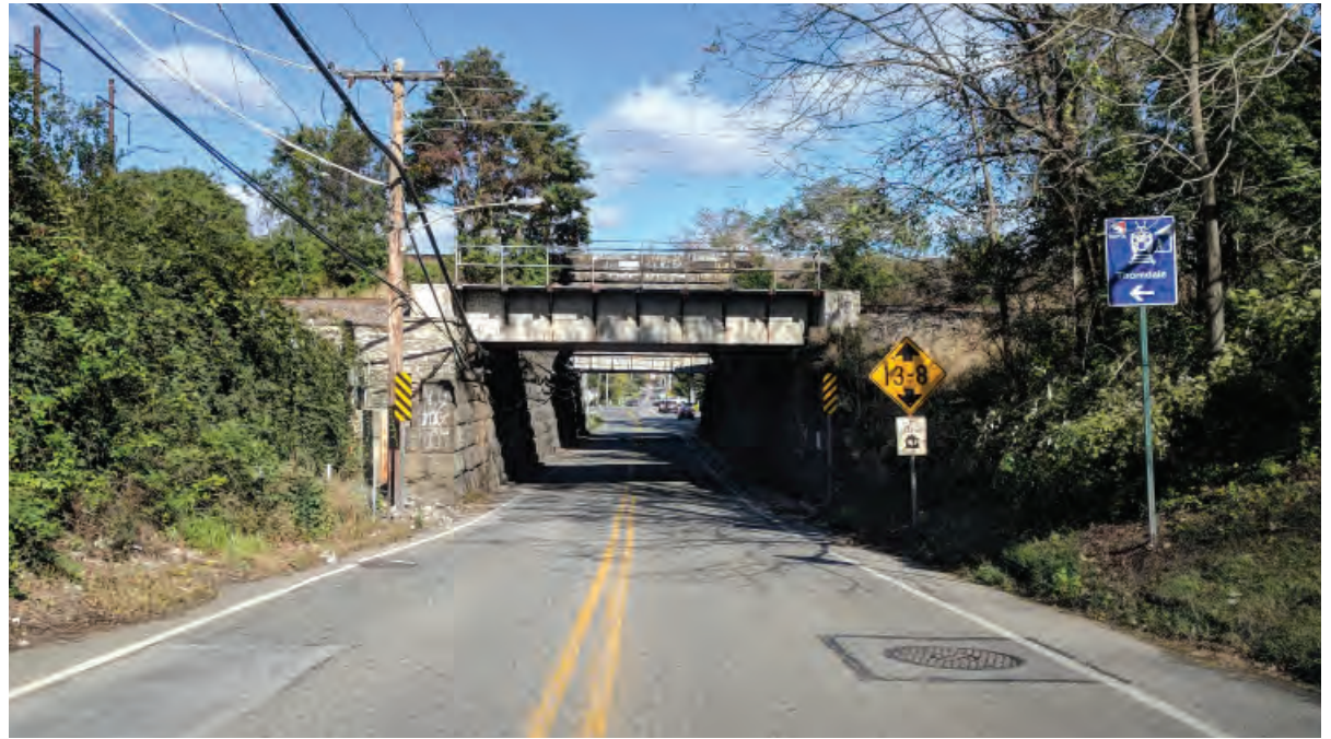
Amtrak overpass over Marshallton-Thorndale Road
