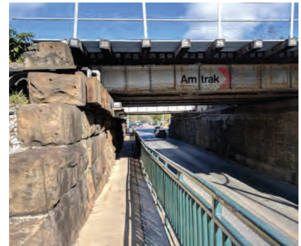
Elevated walkway along Bailey Road crossing under the Amtrak corridor at the Thorndale Station.
