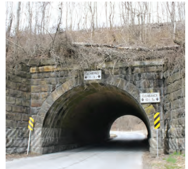
Valley Avenue/Route 372 passes under the Enola Low Grade corridor via this narrow stone arch bridge. Horizontal curvature of the road restricts sight distances at the bridge.
