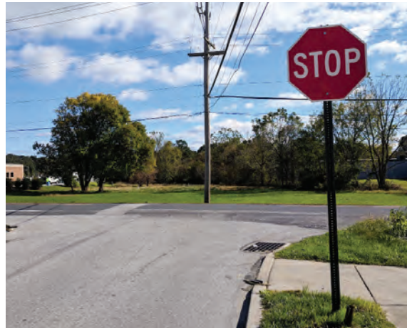
Looking east on Fox Avenue toward the potential future crossing of North Caln Rd.
