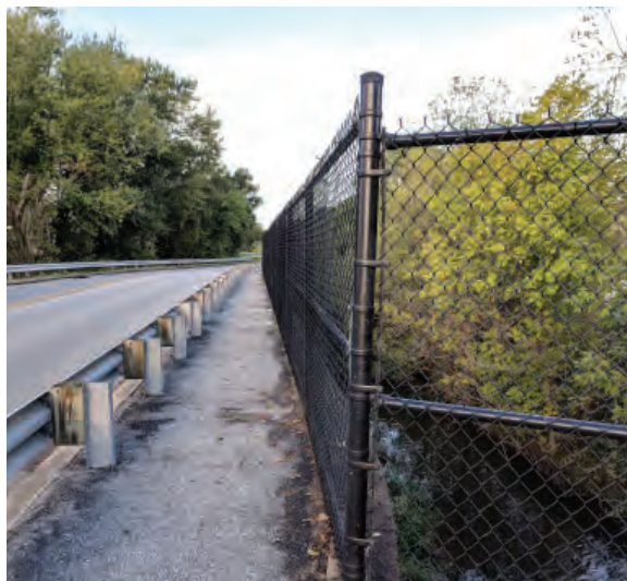
An existing “pinch point” along the GO Carlson Boulevard path
