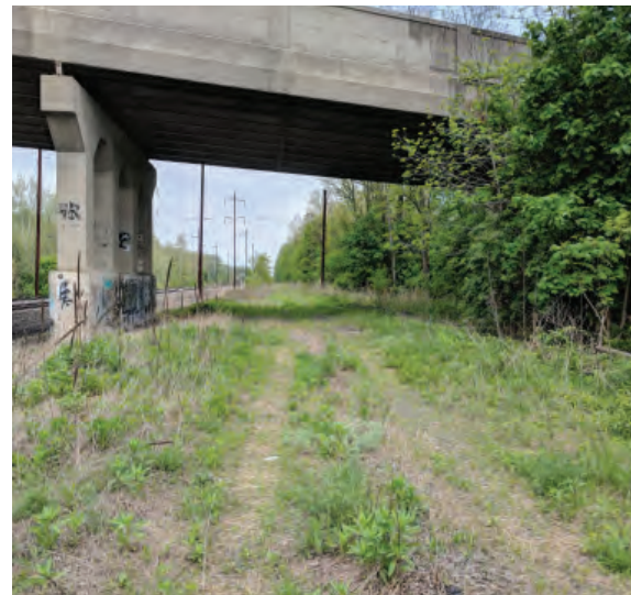
The former Enola Low Grade corridor passes under Route 41.
