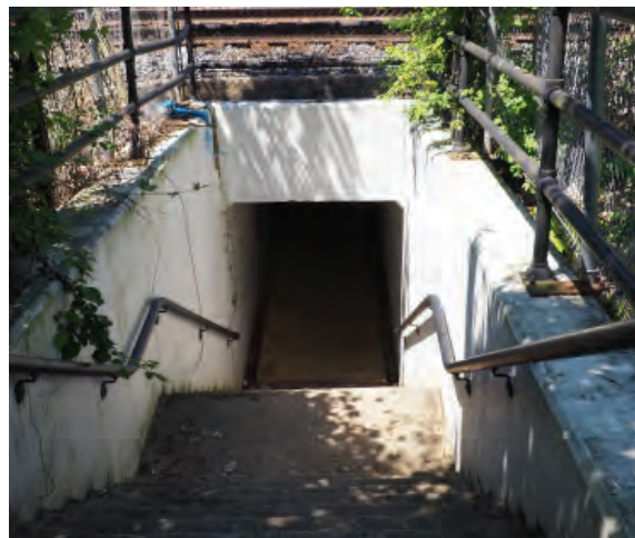
Existing pedestrian underpass under the Amtrak corridor.
